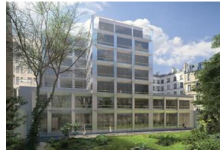
Pre-leasing completed in H1
