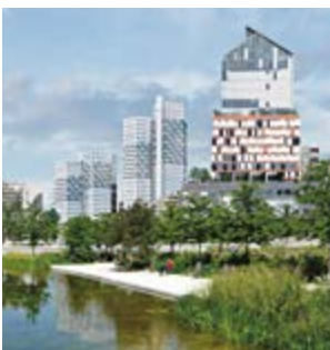
Citylights and Tour Horizons, Boulogne-Billancourt
